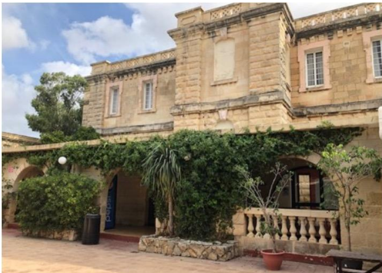
Malta: Language School administration, classrooms below and living accommodation above. Photo: John Sweet
