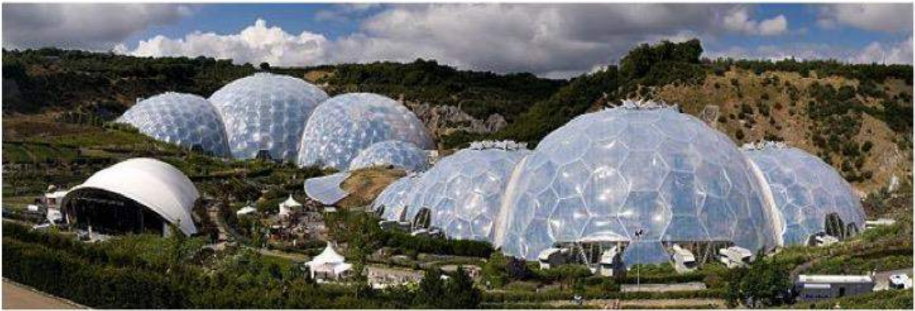
Geodesic domes at the Eden Project: Image by JürgenMatern from Wikimedia Commons
